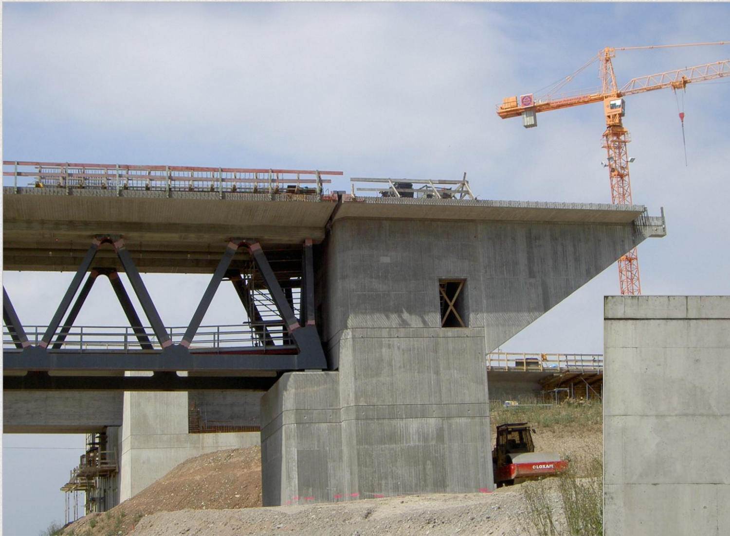
Bridge abutment reinforced concrete
