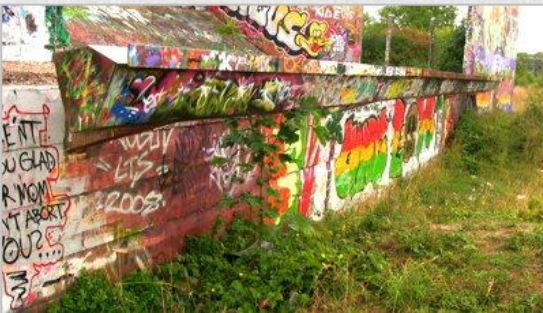
Retaining wall reinforced with concrete
