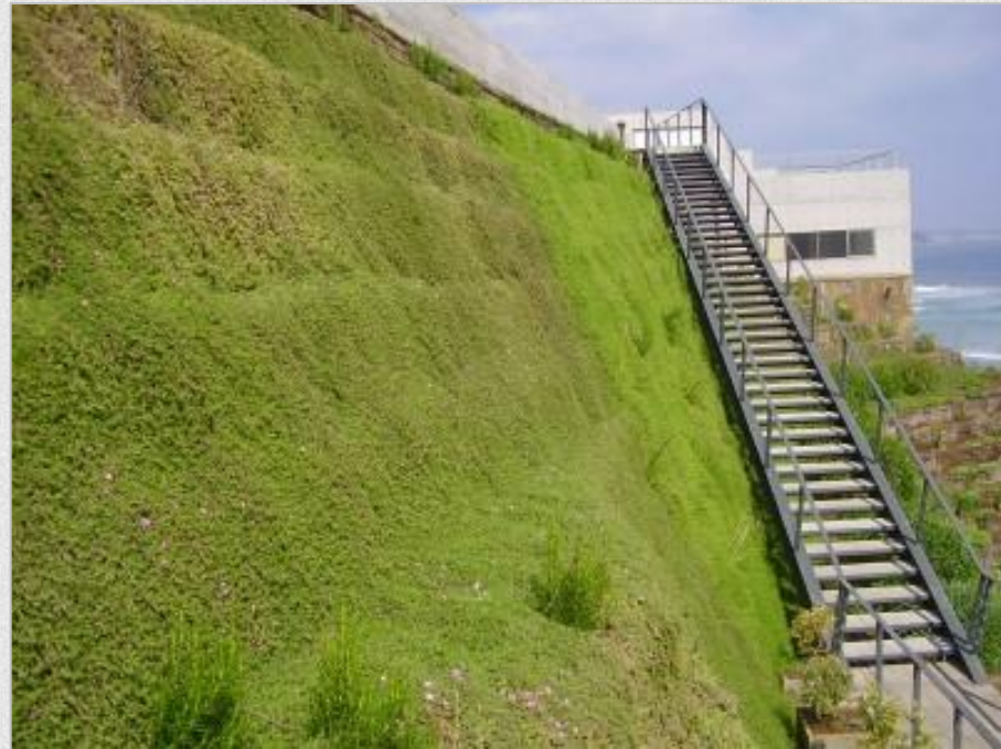
Soil wall reinforced with geosynthetics
