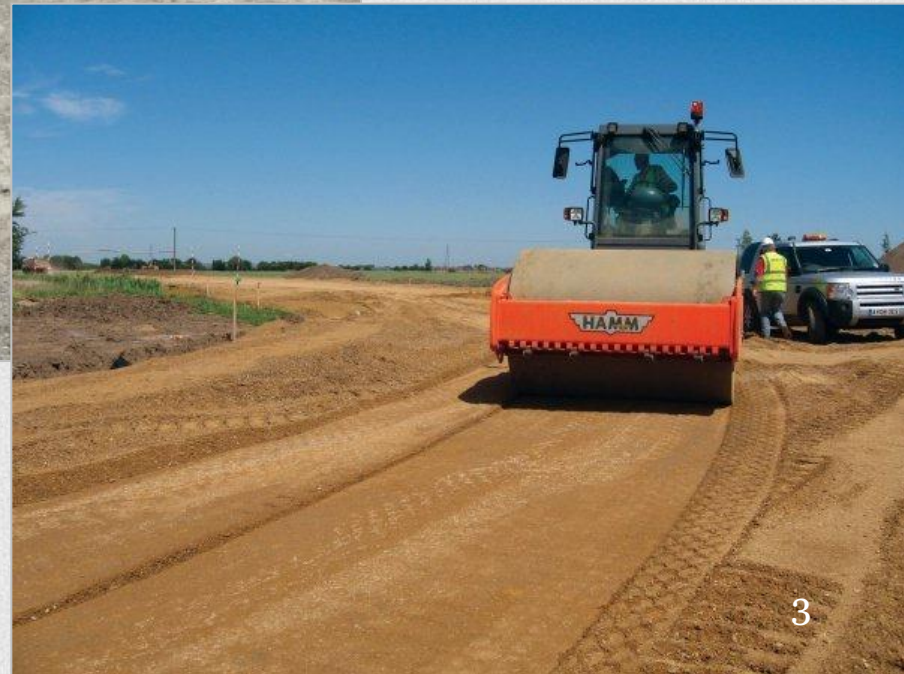
Road Foundation Construction
